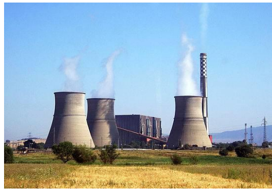
Figure: Cooling Tower
