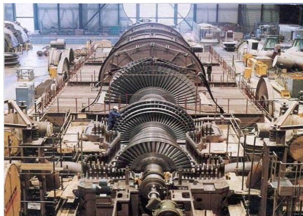
Figure: Steam Turbines
